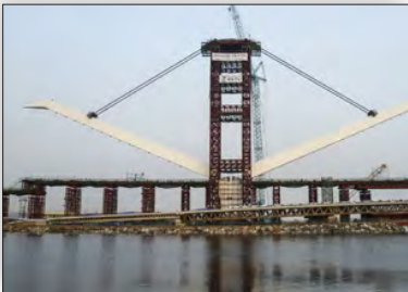
Jacking with high capacity precision control
